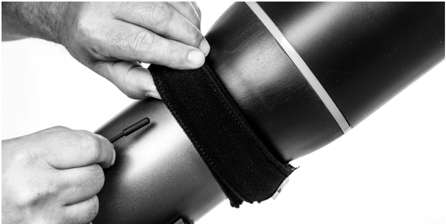
Fig. 1: Place the thermistor under the heating band so that it is secure.
